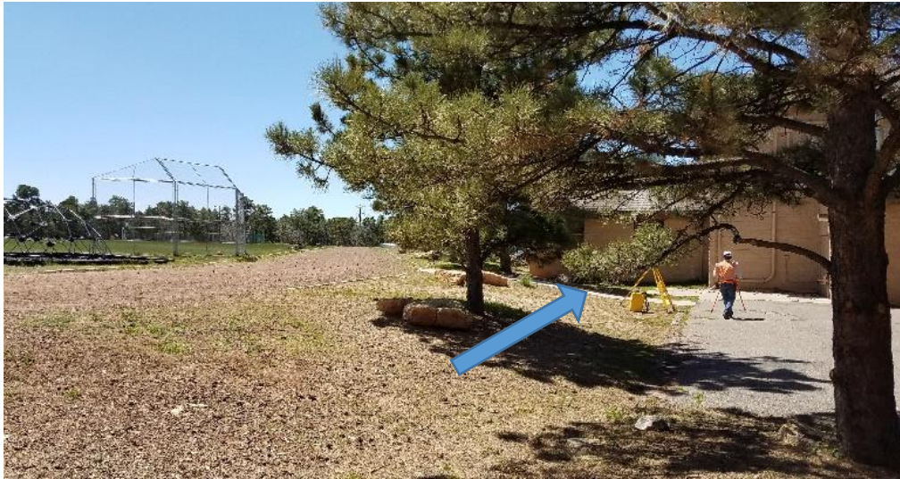
Figure 8: GCHS Building A, problem area 5
