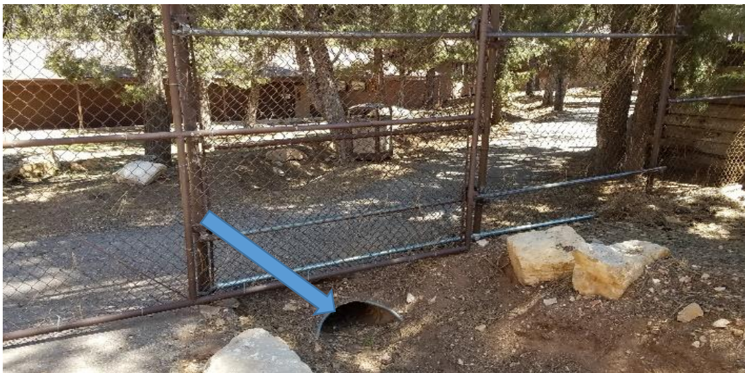
Figure 3: GCHS culvert A
